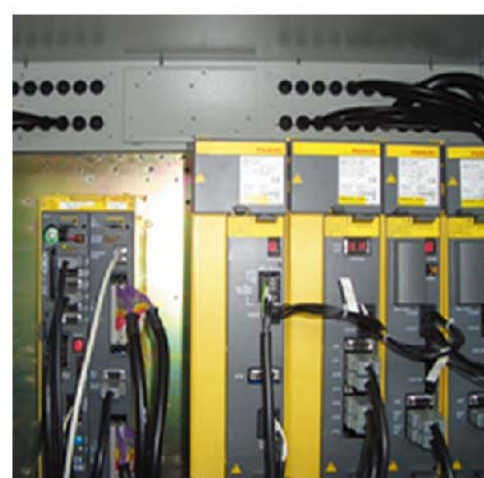
Water-proof fittings are mounted at the openings for wires to avoid invasion of oil mist.
